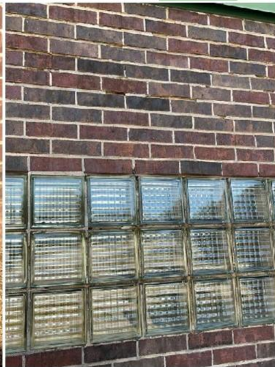
DETERIORATING MORTAR
