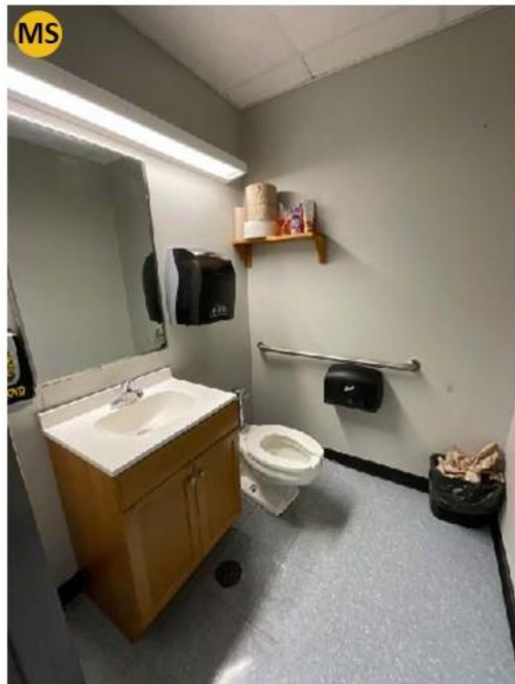
DOES NOT MEET TAS/ADA
