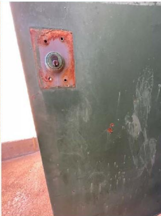
INADEQUATE HARDWARE
