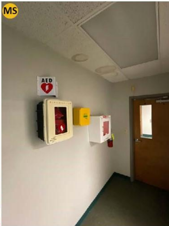
EVIDENCE OF MOISTURE DAMAGE
