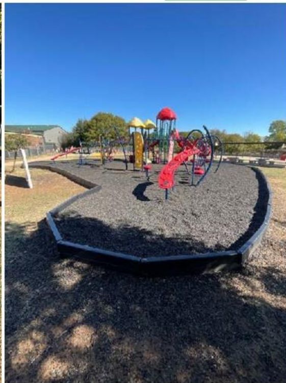
DOES NOT MEET TAS/ADA
