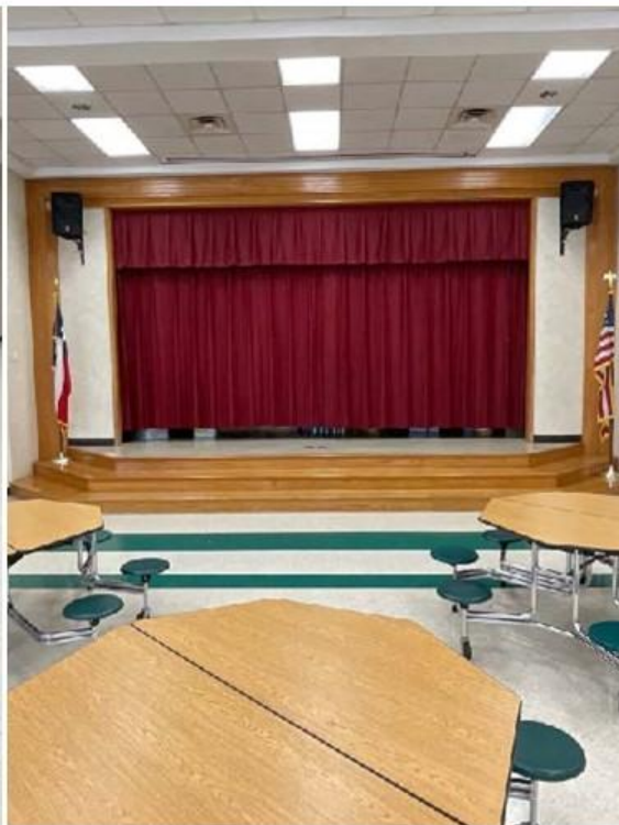
DOES NOT MEET TAS/ADA
