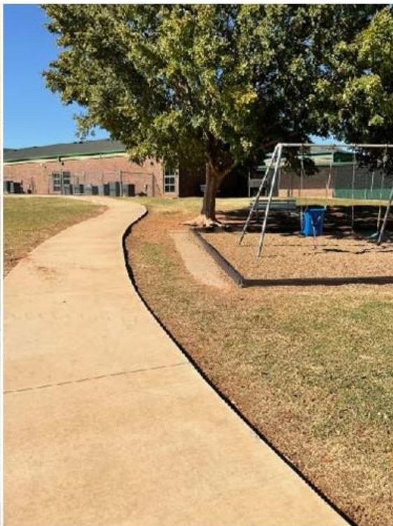
DOES NOT MEET TAS/ADA
