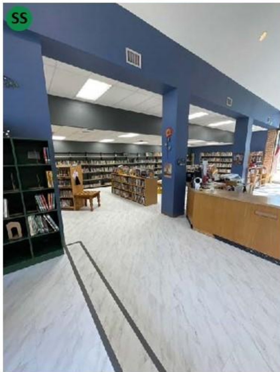
DOES NOT MEET TAS/ADA
