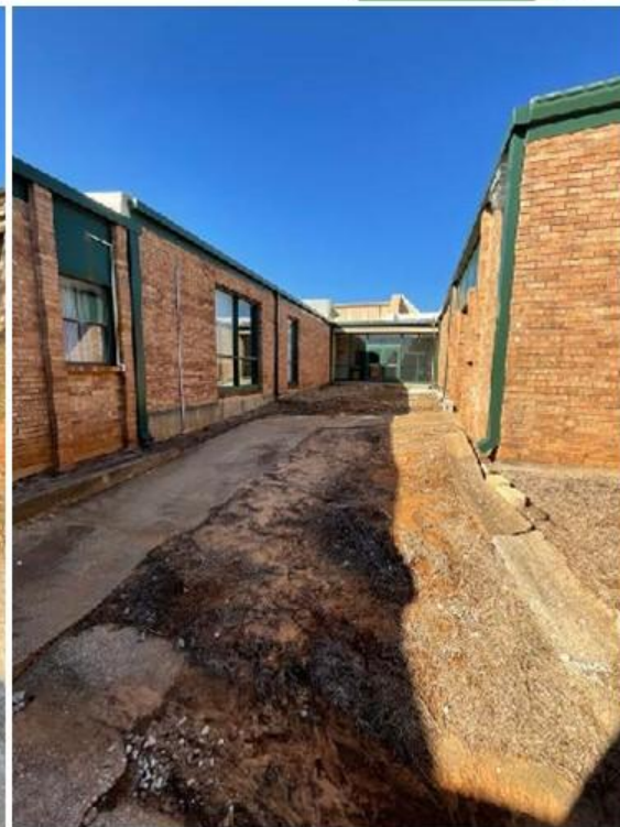
INADEQUATE DRAINAGE
