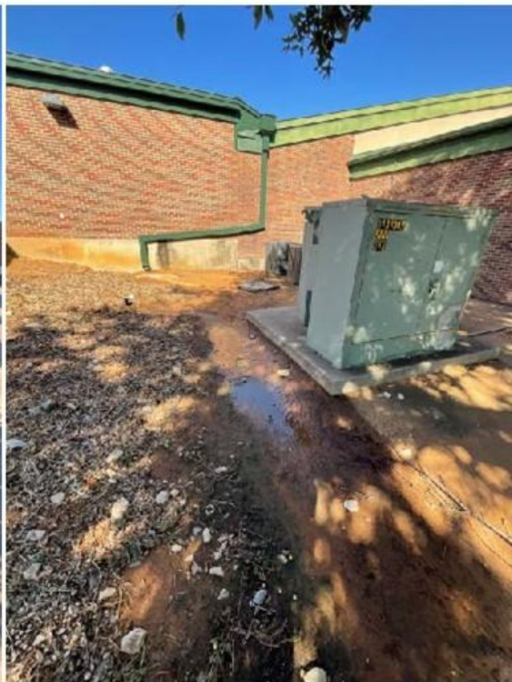
INADEQUATE DRAINAGE
