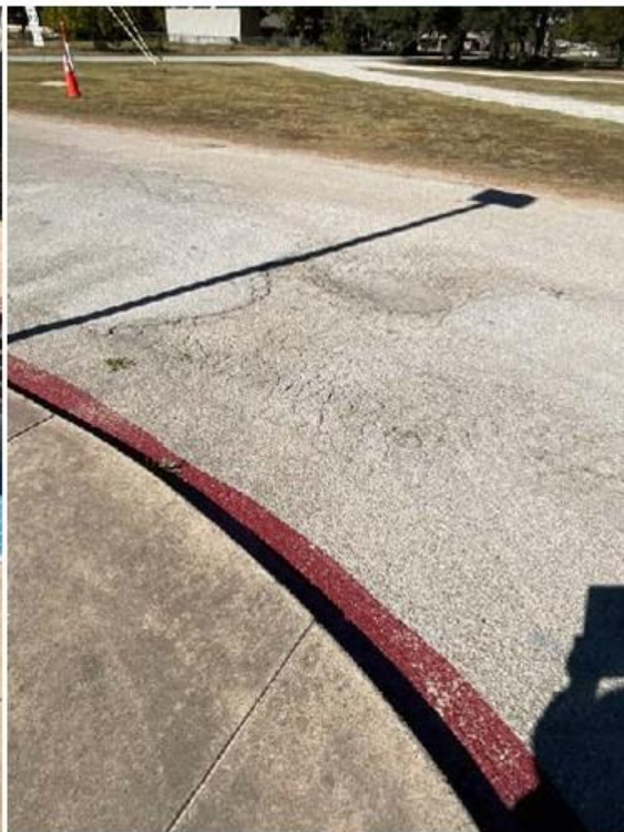
DETERIORATING PARKING/STRIPING
