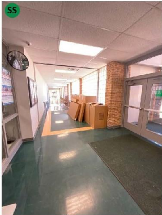
NEEDS SECURE VESTIBULE
