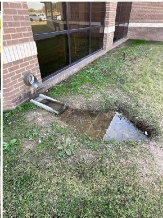
INADEQUATE DRAINAGE
