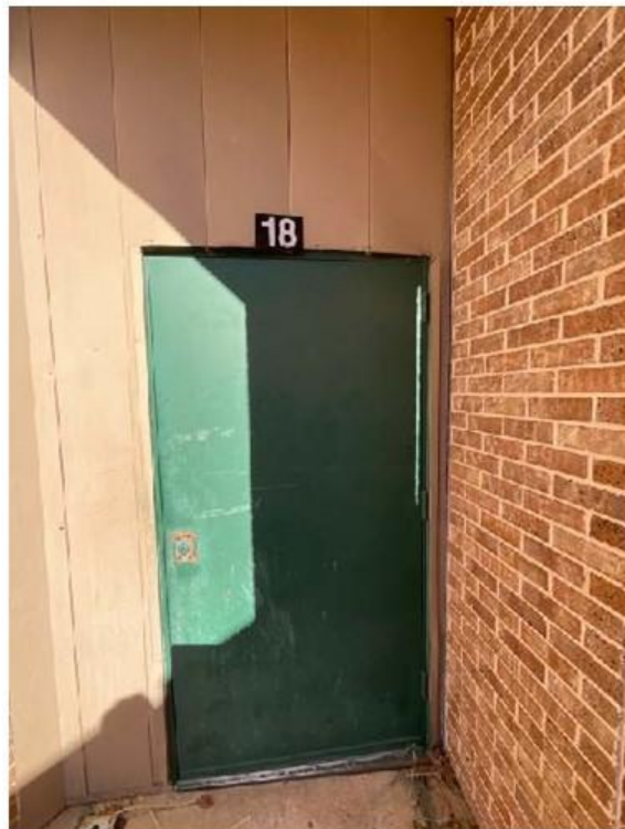
INADEQUATE HARDWARE
