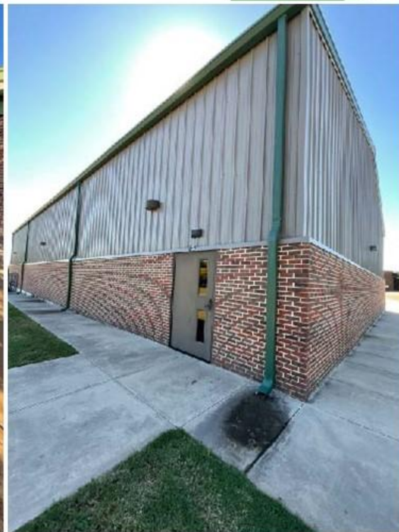
INADEQUATE DRAINAGE
