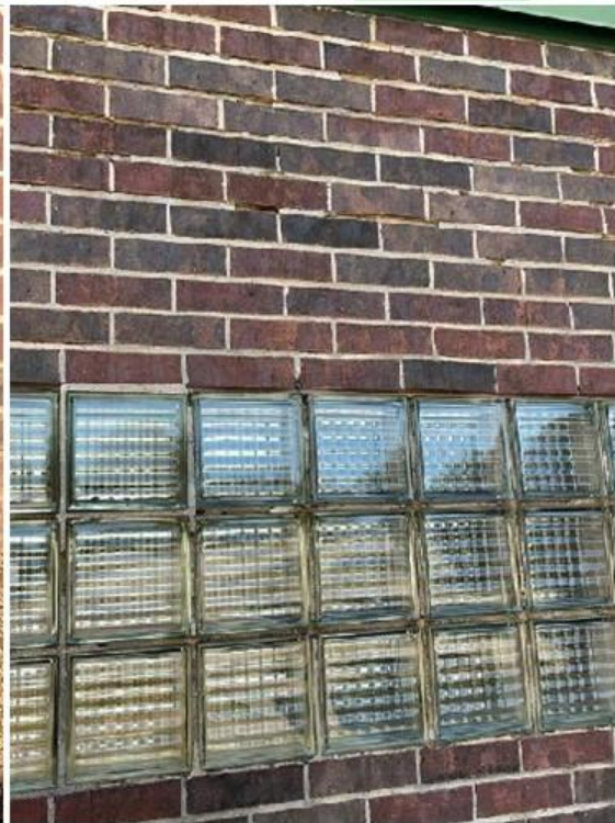
DETERIORATING MORTAR
