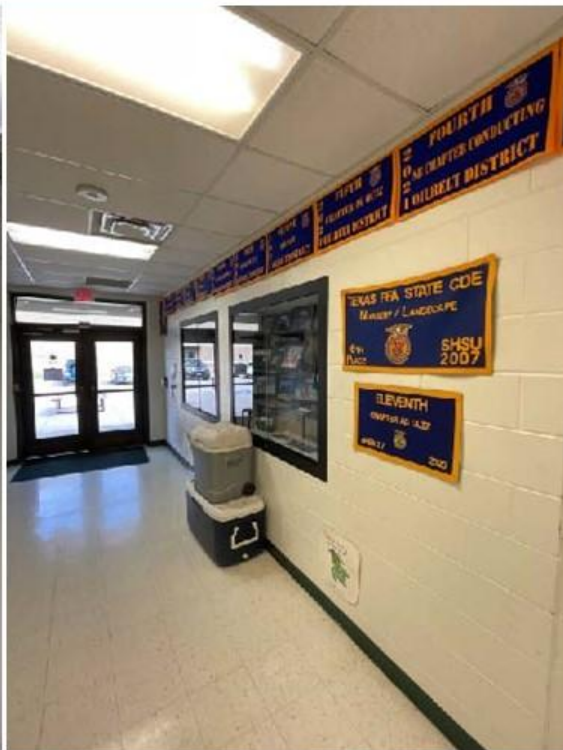
NEEDS SECURE VESTIBULE
