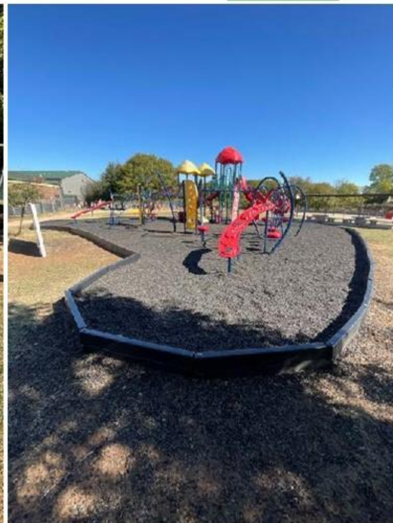
DOES NOT MEET TAS/ADA
