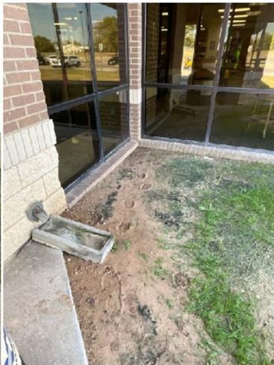
INADEQUATE DRAINAGE
