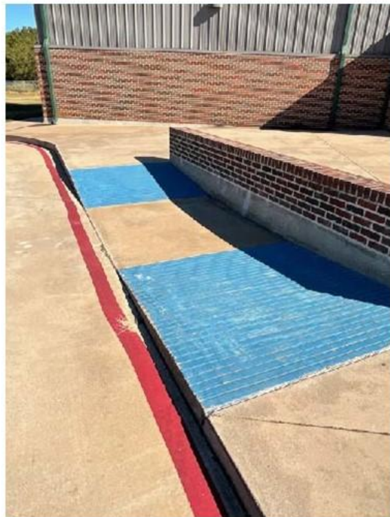
DETERIORATING PARKING/STRIPING
