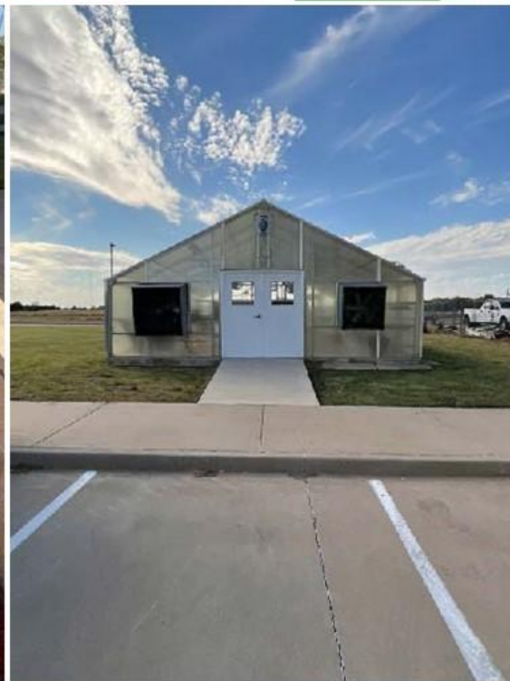
DOES NOT MEET TAS/ADA
